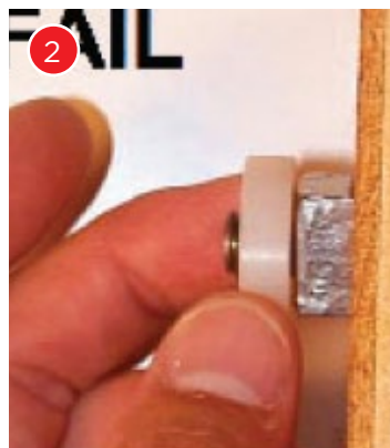
This bolt end is an unsafe protrusion.
